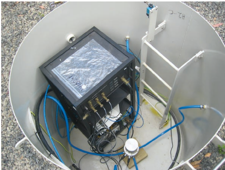
Fig. 2.4 Photograph showing the interior of an array element equipment vault at IS04 Shannon, Australia
